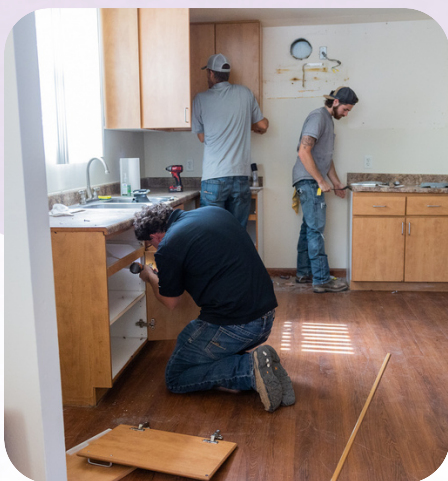
Updating our Transitional Housing apartments with new cabinets and countertops
